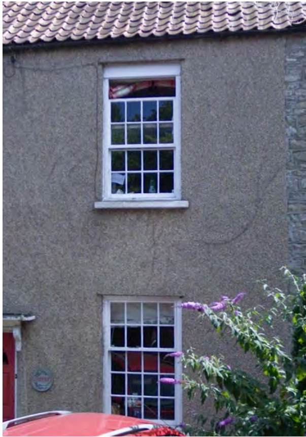
Vandyck Avenue: A few examples of the original format of Georgian windows survive around the Conservation Area.
