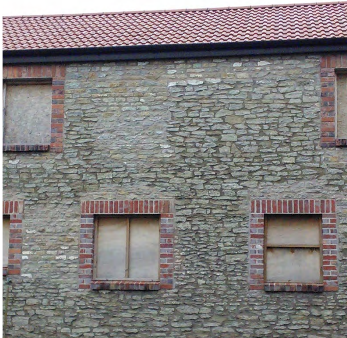
Dapps Hill, Avon Mill Lane, Wellsway, Chew Park: Brick edging to rubble stonework is a noticeable feature around the Keynsham Conservation Area.
