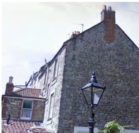
Dapps Hill: Brick chimney stacks emerge from rubble stone gables and rubble building walls.
