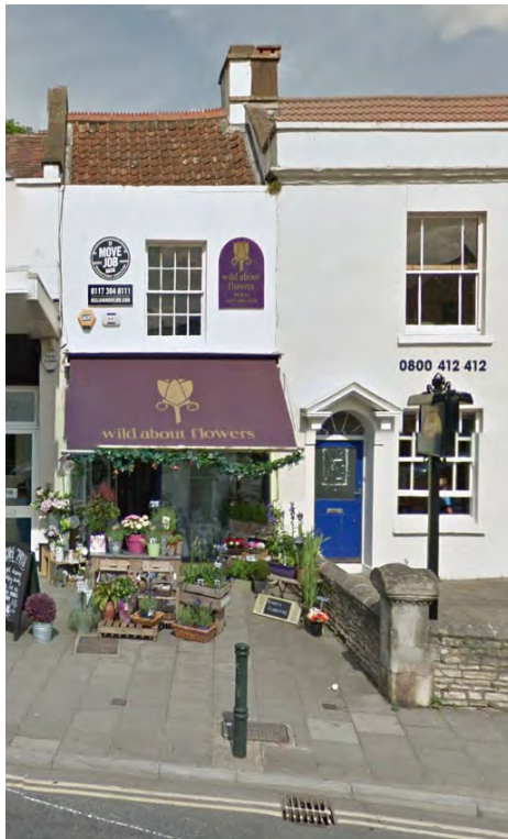
High Street: Some plot widths are narrow, accentuating the vertical emphasis of building frontages. Low coped stone rubble front boundary walls are often terminated by dressed stone piers with sometimes elaborate capitals.
