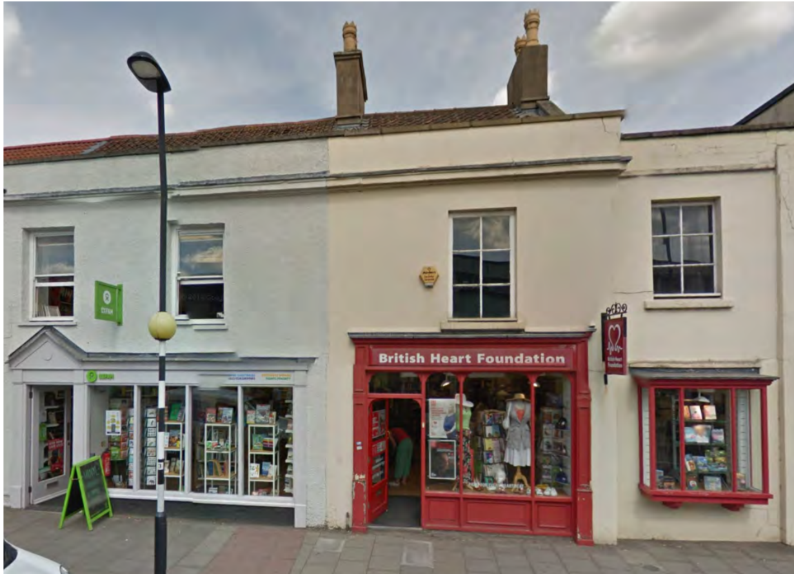
High Street: Traditional shopfronts with signage that is not over-sized. Traditional hanging signs. A cornice runs below the parapet with overhanging coping, articulating the top of the walls. Subdivisions between properties punctuated with chimneys and some gable parapets, subdivisions also accentuated by subtle changes of paint colour.
