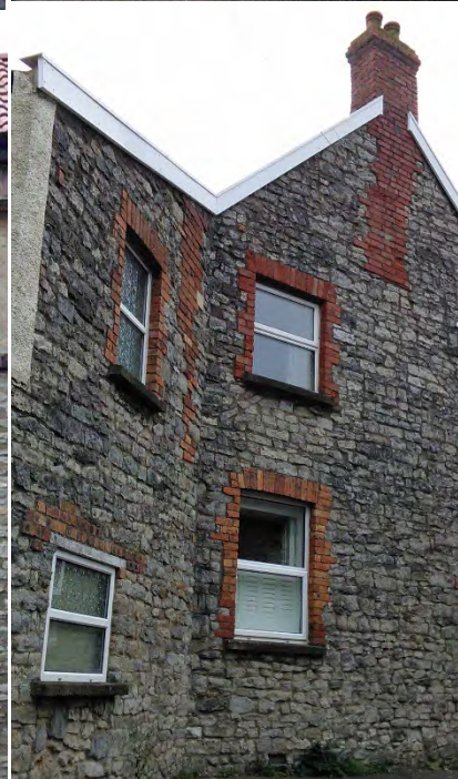
Dapps Hill, Avon Mill Lane, Wellsway, Chew Park: Brick edging to rubble stonework is a noticeable feature around the Keynsham Conservation Area.
